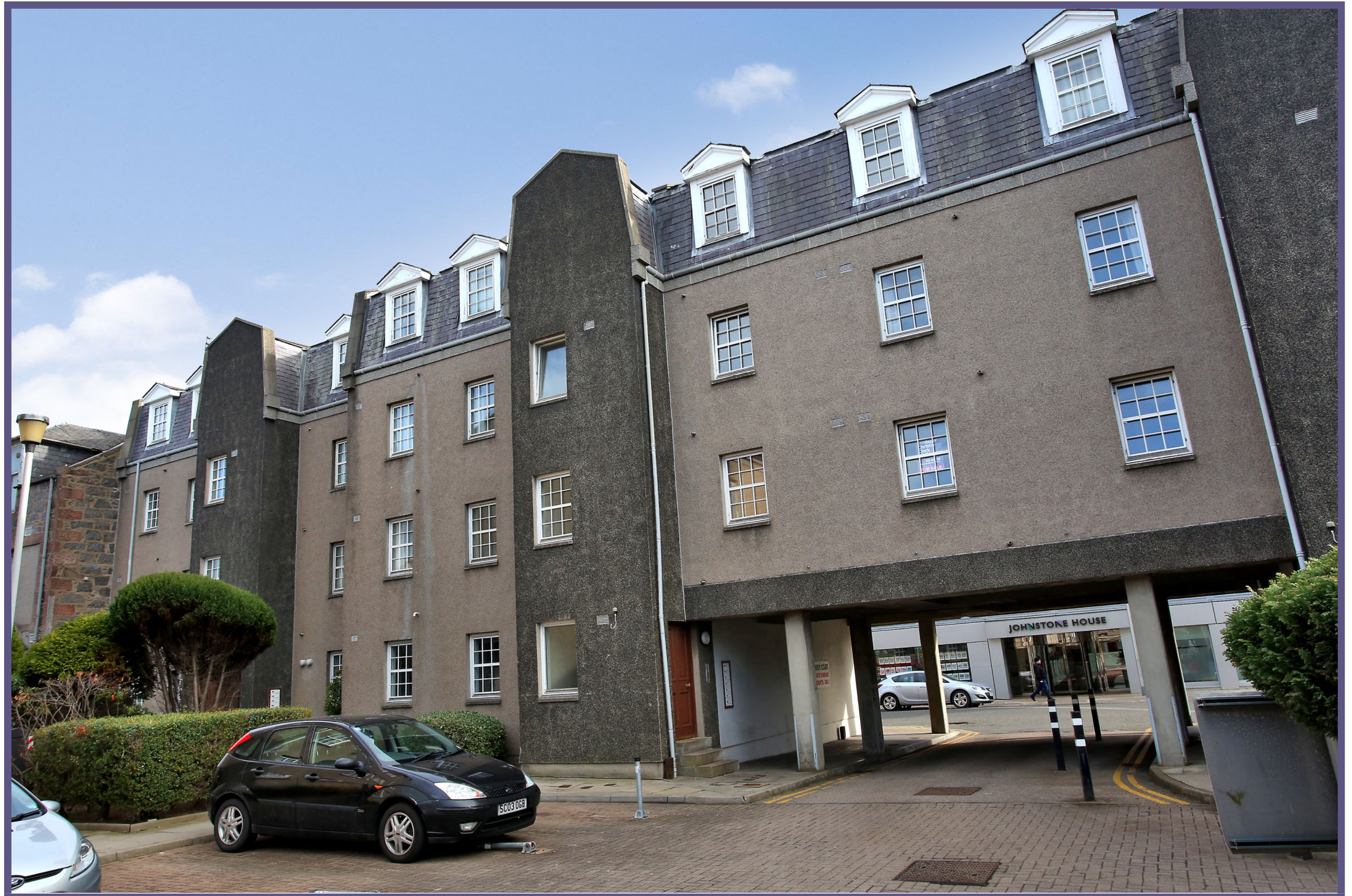
Entrance to Courtyard
